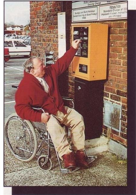
**Barrier Controls** - Manual controls, the coin entry slot, and the ticket issue on barrier control units should be between 1000mm and 1300mm above the ground, as required by BS6571:Part 4:1989. Instruction plates should be placed at the lower end of the range (1000mm to 1600mm above the ground) required by the Standard.
