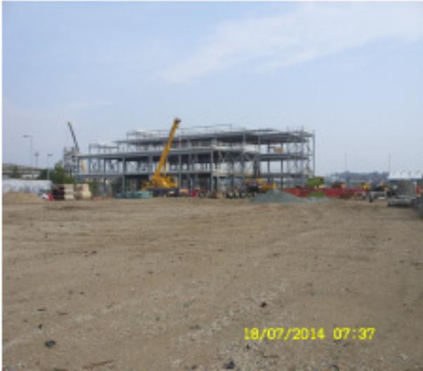
**Photo 1**-View from the Southern most point of the site with all pre cast planks now in place and drainage works to car park now commencing.
