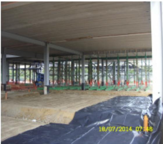
**Photo 6** – North side ground floor slab showing DPM being laid in preparation for reinforcing bars.
