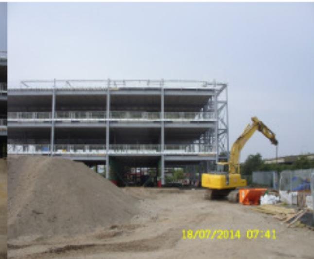
**Photo 4**-View from North of the steel frame with all pre cast floor now in place
