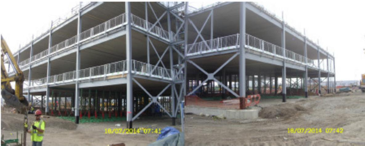
**Photo 5** – View looking East at the showing all planks now in place
