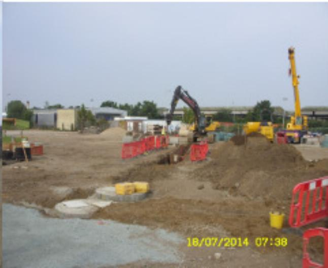
**Photo 2** -View from the East showing all deep drainage works working towards one of the petrol interceptors
