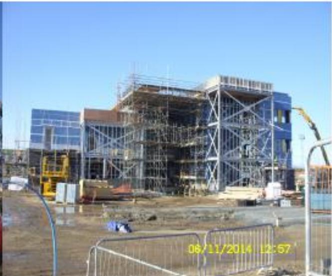
**Photo 2** – View from the East, large birdcage scaffold in the foreground to be used to construct the entrance canopy.
