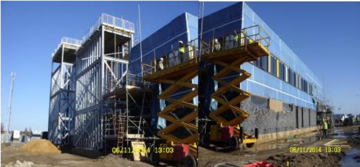
**Photo 5** – View looking South East showing framework to Fire escape stair 1 and 4 ready to receive Trespa cladding
