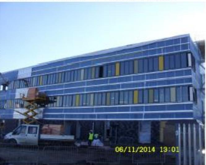
**Photo 4** – View from the North, showing ribbon windows and rain screen cladding in progress.
