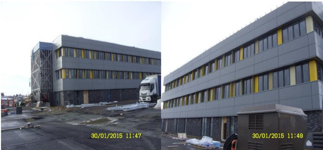
**Photo 3** – View from the North side of Riverside Road, showing Trespa framework to fire escape stairs
