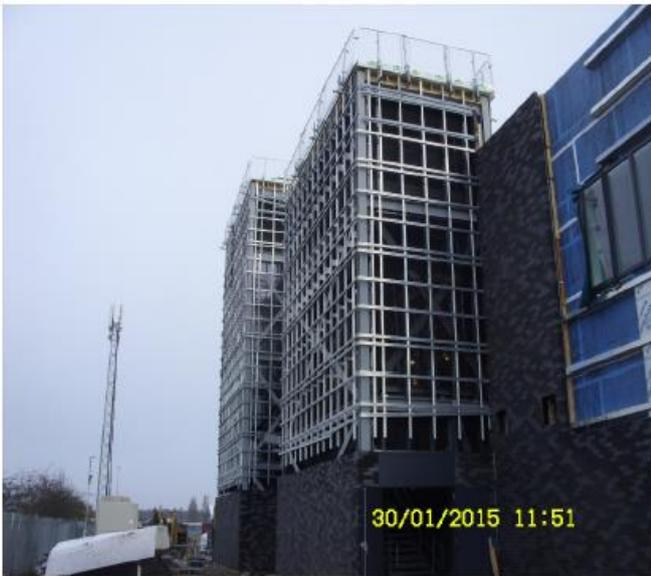
**Photo 5** – View looking South East showing brickwork now complete, and framework ready to receive Trespa cladding.
