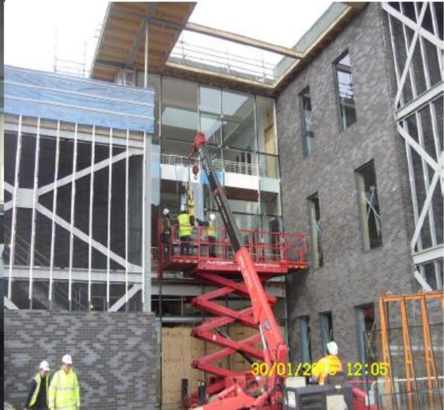
**Photo 8** – View showing glazing being installed into East curtain wall
