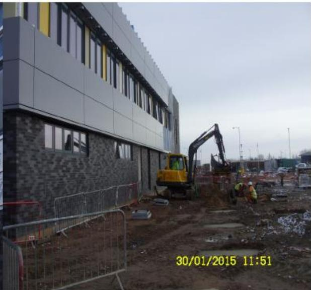
**Photo 6** – View looking East on South Elevation, showing groundworks casting cycle shelter bases
